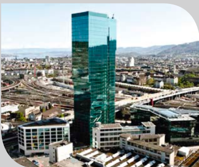
Prime Tower, Zürich*
